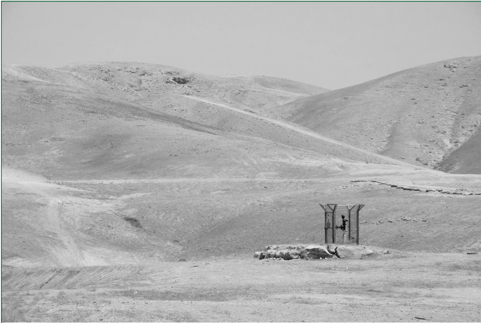
Mini station of the water pipeline in Negev desert in Israel. The ever-present extreme water scarcity in Israel has led to the continuous development and adoption of creative technologies and institutions.
